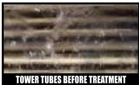
TOWER TUBES BEFORE TREATMENT
