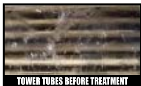
TOWER TUBES BEFORE TREATMENT
